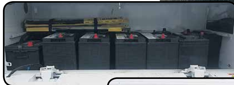
Reinforced shelf carries 10 batteries.
